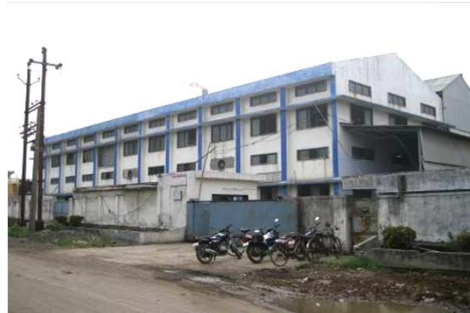
Plant buildings with gates and guard post
