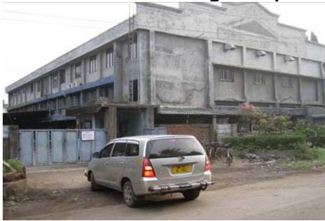
Plant entrance with gates and a guard post
