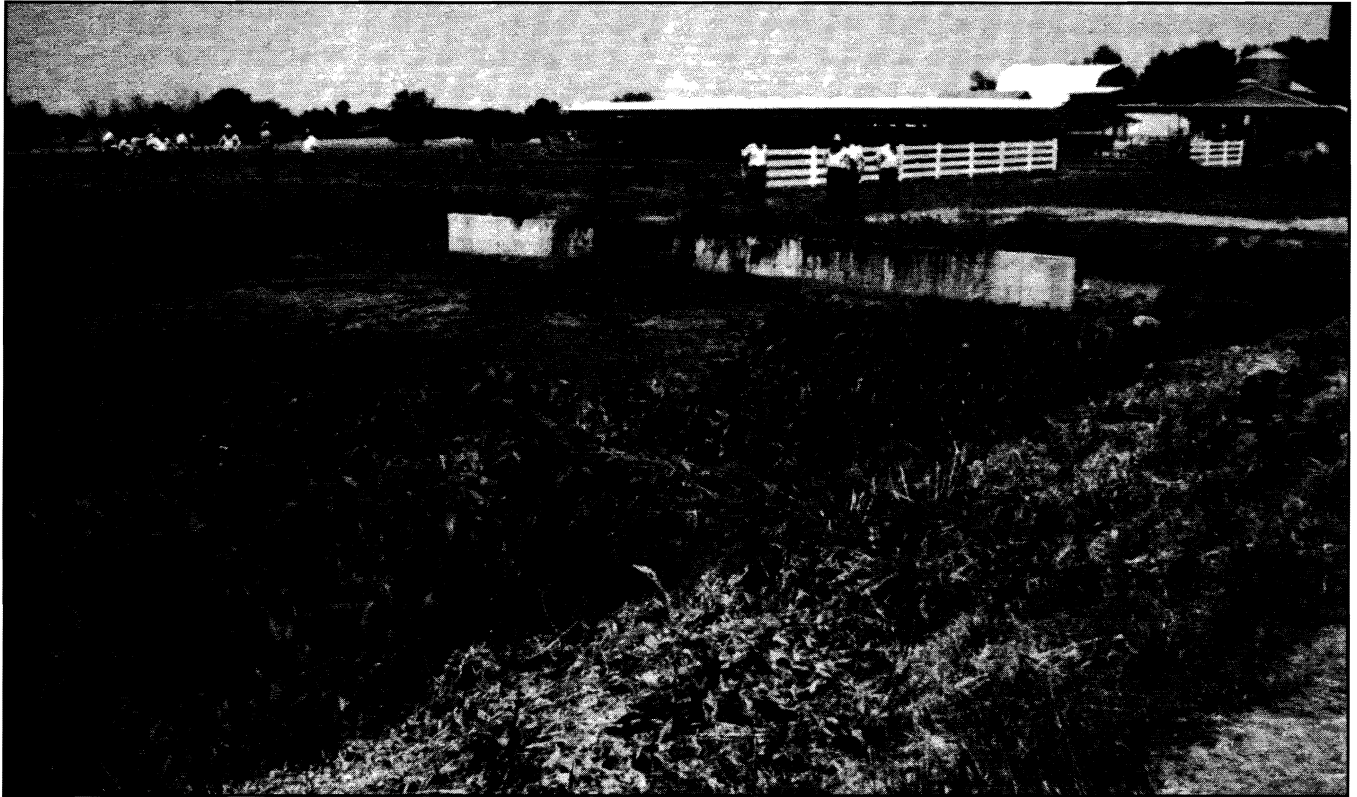
Overgrown pit due to no agitation.
