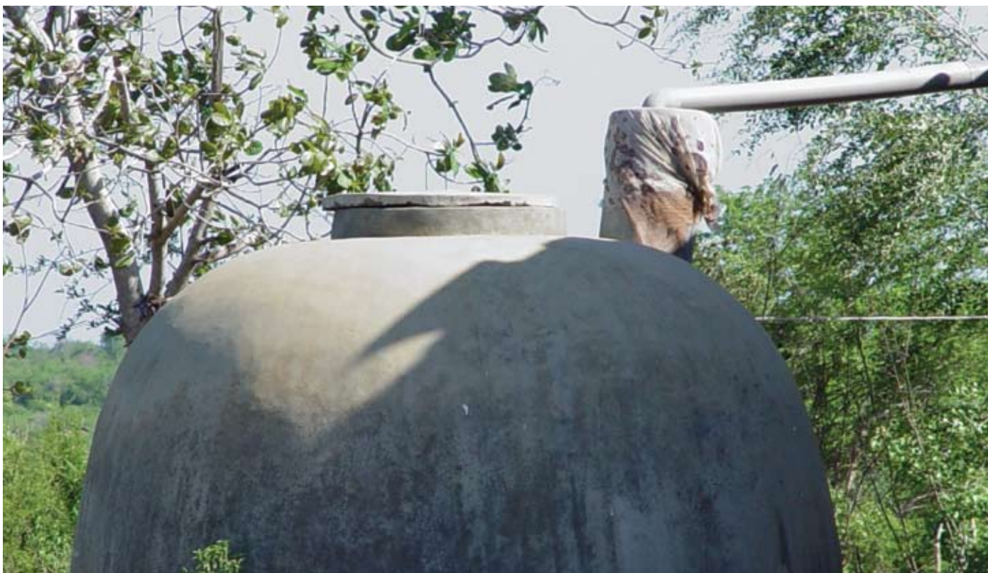
Providing rainwater harvesting systems (like the water storage tank pictured here) to households in drought-prone areas can help communities adapt to the challenges of future climate change.
