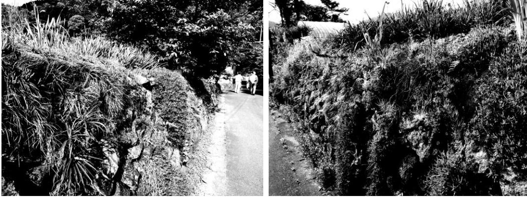
Image 6.4.3.3: Rock retaining walls in Kabu shuraku (left and right)
