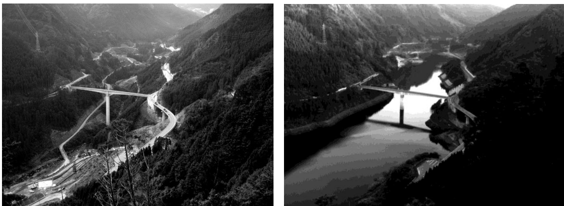
Images 6.5.4: Oyama Dam construction, Feb 2008 (left) and completed, May 2012 (right)
