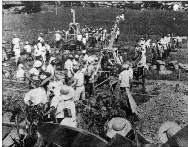
Image 4.3.5.1: Community members build cable broadcasting infrastructure
