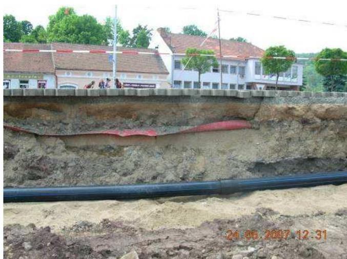
Figure 11 - An example of anthropogenic layers formed of gravels, sands and loams at Oslavany Square near Brno, Czech Republic, where a water pipeline is laid (Photo courtesy of L. Svoboda).
