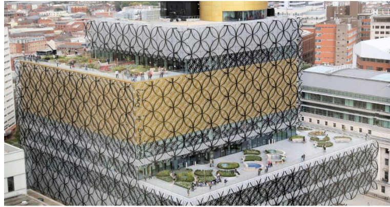
Birmingham Library Rooftop Garden
