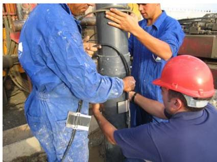
Fig 3. Attaching downhole electrodes to borehole
