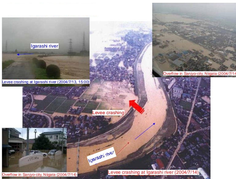
Figure 2 Levee crashing by 2004 Niigata torrential rainfall at Igarashi river, July 2004 (Photos is from the Hokuriku Regional Bureau, Ministry of Land, Infrastructure and Transport in Japan).
