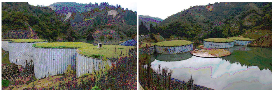
Figure 11 Debris barriers made by disaster wastes which were generated by 2004 year Niigata Chuetsu earthquake.
