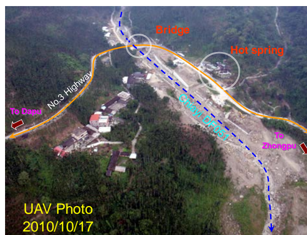
Fig. 6 UAV photo of Chiayi DF051 torrent after Typhoon Morakot
