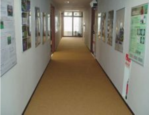
(c) Corridor installed IC Tag Textile Carpets
