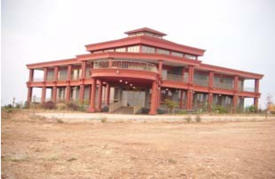
Figure 7: The new rehabilitated structure of the Igence Palace, 2012
