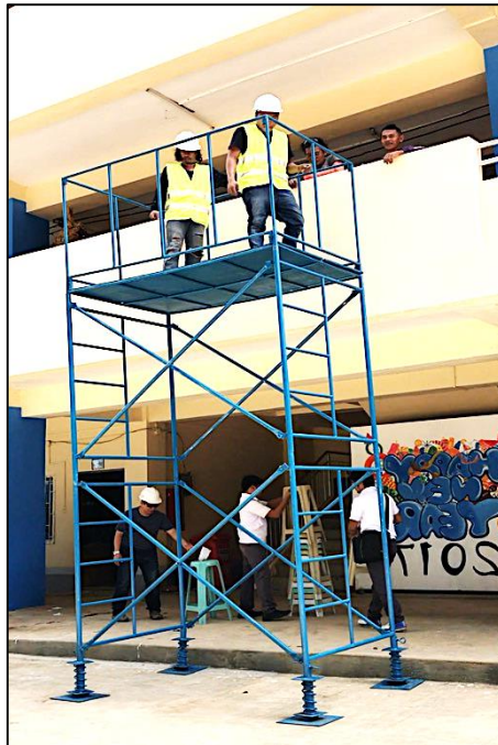
Figure 9. Actual Photo of two storey scaffold in an incline Plane
