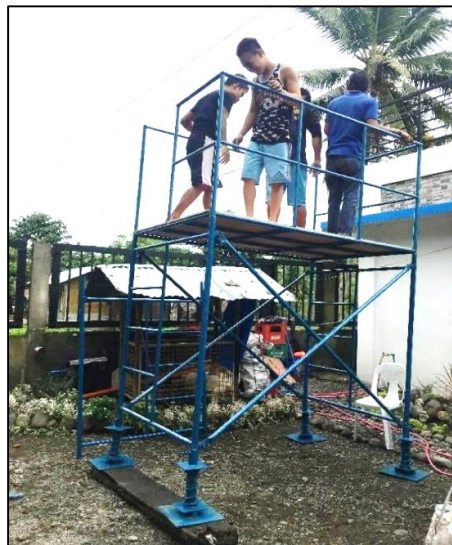
Figure 7. Actual Photos of One-Storey Scaffold on a Flat and Irregular Surface
