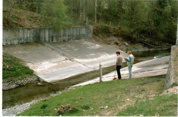
Plate 1 Trapezoidal flume on the River Dulas at Rhos-y-pentref
