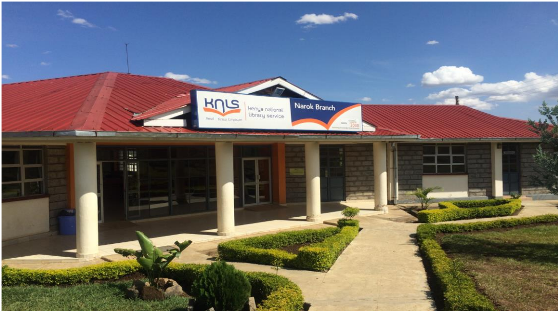
Photo 3: Narok Library building
