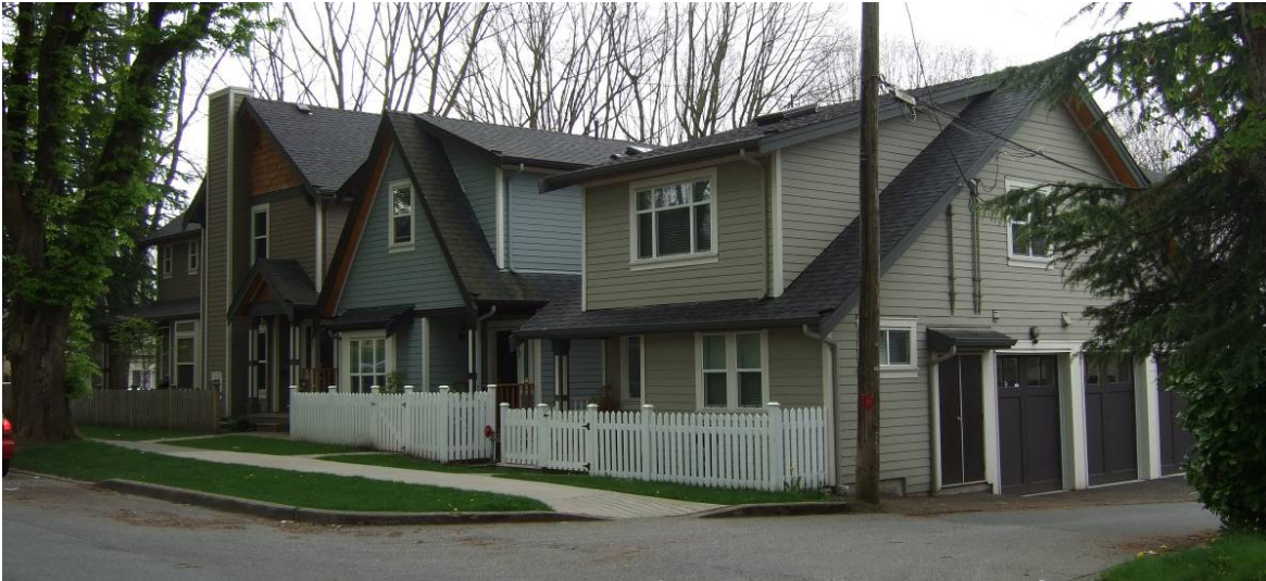
Figure 18: 1099 East 21st Avenue – Duplex and Small House (9)
