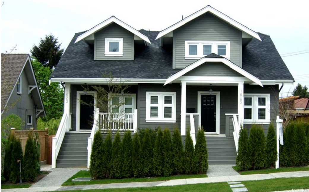
Figure 12: 1621 East 21st Avenue – Character Retention and infill (3)
