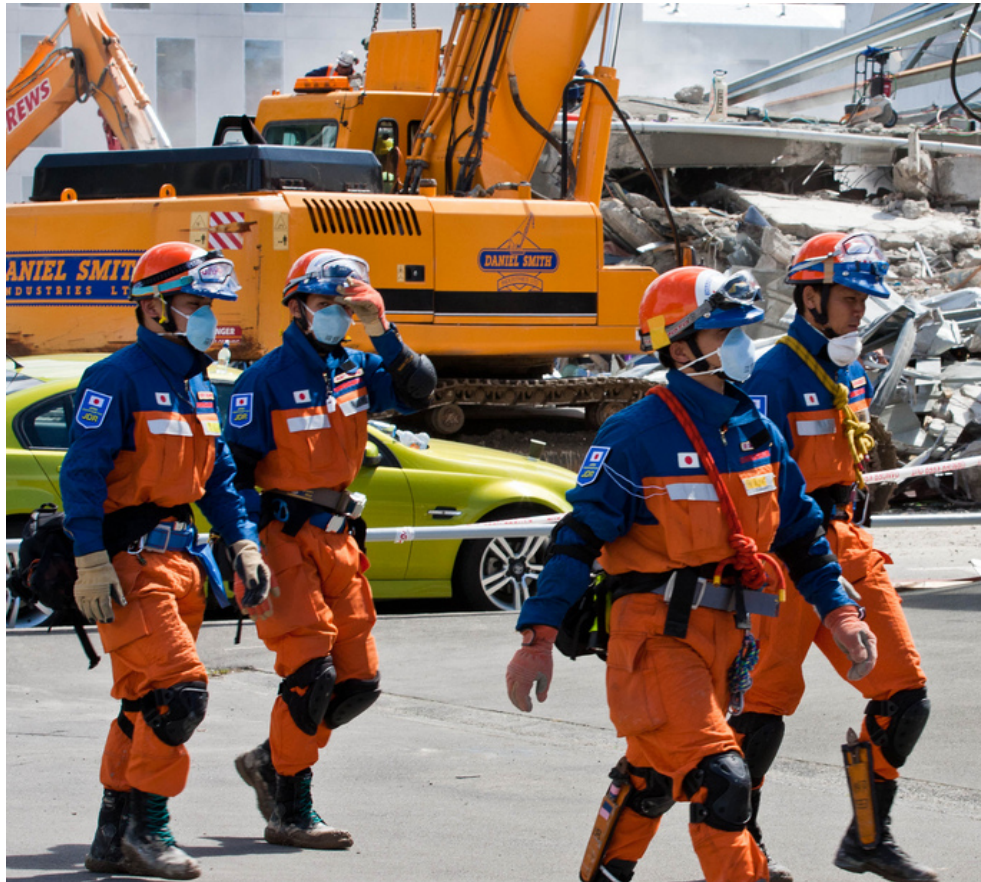
Figure 3. A Japanese urban search and rescue team at the ruins of the CTV building, Christchurch, 24 February 2011 (Gabriel, 2011).
