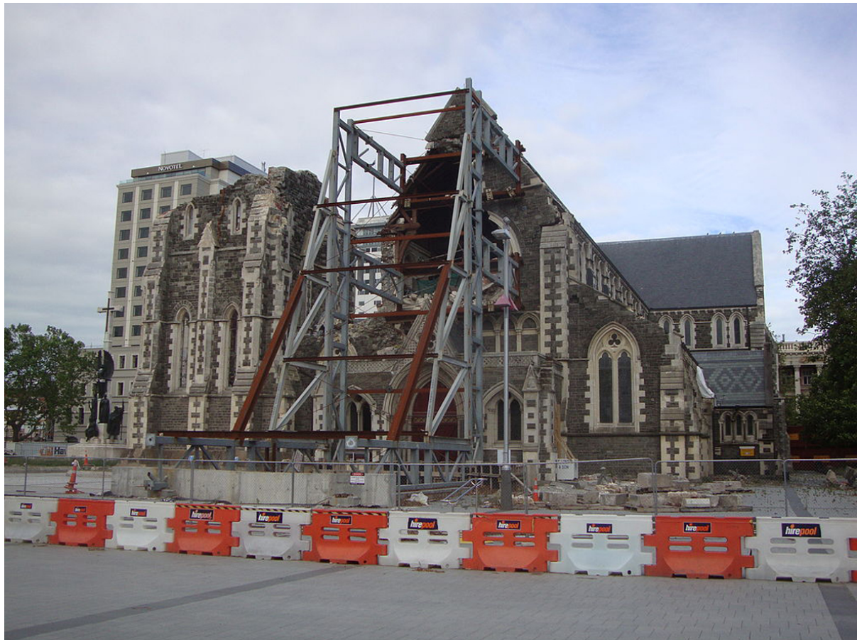
Figure 1. Christchurch Cathedral just before the December 2011 earthquake (Schwede66, 2011).
