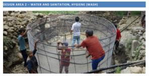
Fig. 7. Constructing a new rainwater tank in Sandikohla, 2013
