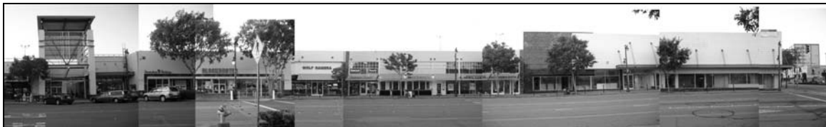
Fig.26 View of the rest of the north elevation of the proposed site. The property along El Camino Real (at the right edge of the photo) is currently vacant. (Source: Author's files)
