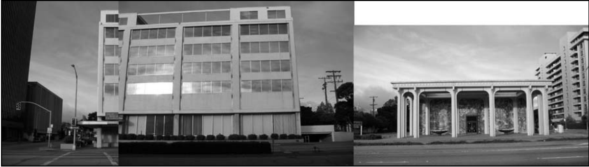
Fig. 34 Two buildings along El Camino Real, northwest of the site. The bank building on the right is particularly sculptural in form, but is placed too far back (about thirty feet) from the street. (Source: From Author's files)
