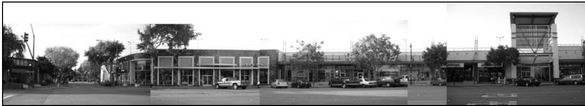
Fig. 25 View of the north elevation of the proposed site, along Fourth Avenue. Shown here is half of the elevation of the retail strip. The street at the left is San Mateo Drive. The glass canopy on the right signals an atrium which leads to the parking lot on site. (Source: Author's files)
