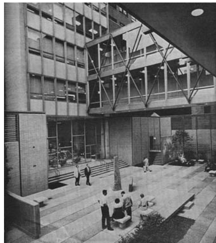
Fig. 59 Atrium space of the New School for Social Research. (Source: Vogelgesang)
