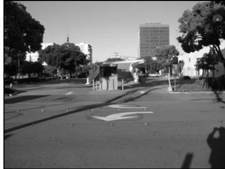
Fig.28 Another view of the unsightly parking ramp (Source: Author's files)
