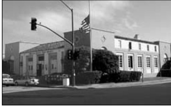
Fig. 15 210 South Ellsworth (Post Office) (Source: www.ci.sanmateo.ca.us )
