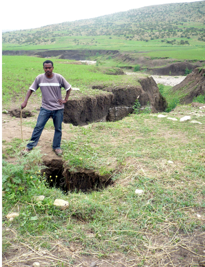
Fig. 1. Gully erosion initiated by soil piping in a Vertisol near May Mekdan (see Fig. 2, August 2010). The soil pipe inlet is located directly in front of the person standing and connects to the 4 m deep gully in the background.
