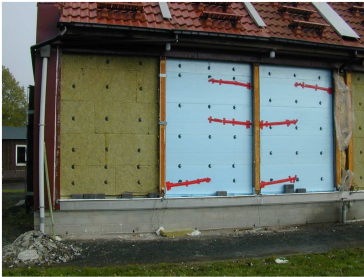
Measurement equipment at different heights and different interfaces in the building components.
