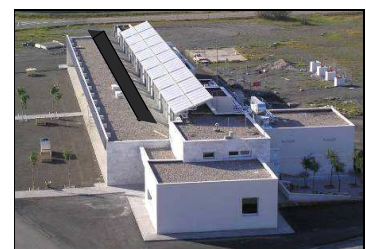
Office building in use.
