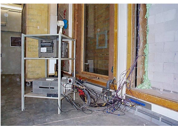
Data logging of the building elements: all sensors are connected to the logger via plug-in-cards.
