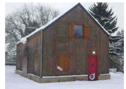
Blower-door test conducted on the building
