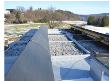
Investigation regarding roof shadings
