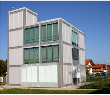
South-west view of the VERU test building.
