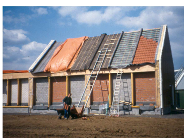
Picture during construction of building elements: the measurement bays with fill in masonry for test walls and the construction of test roofs are visible.
