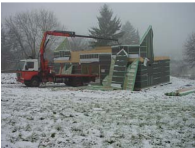
View of the facility during construction
