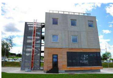
Eastern façade of KUBIK
