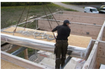
Mounting of roof assemblies
