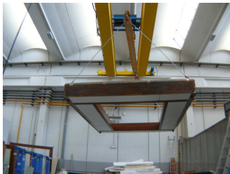
Installing the insulation frame for roof samples in ILARGI.
