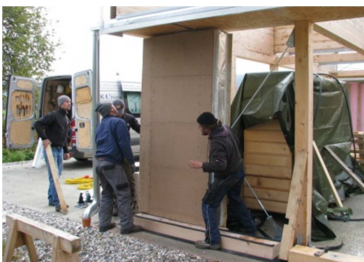
Mounting of wall assemblies
