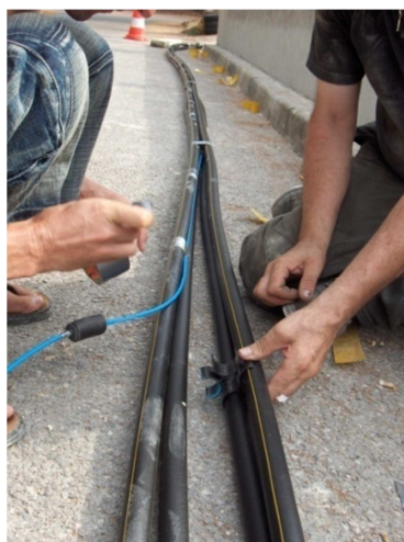
Integration of thermocouples in the double-U ground heat exchanger
