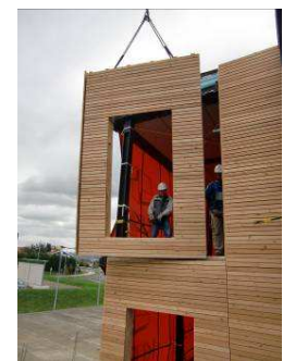
Wooden façade element, developed together with Biohaus Goierri, S.L.
