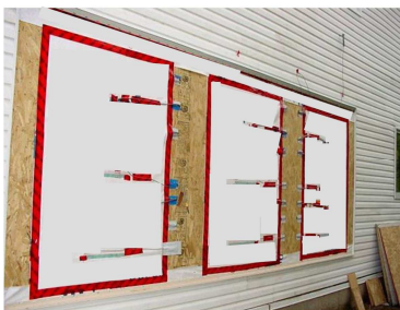
Test bays nearing completion.
