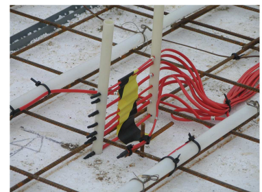
Embedded temperature sensors in the floor of one of the side-by-side test rooms in EnergyFlexLab before concrete was poured in.
