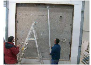
Samples are constructed under controlled conditions inside the pavilion.
