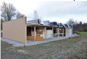
Facility during erection process
