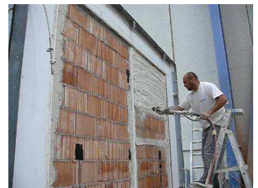
Insulating mortar projection.
