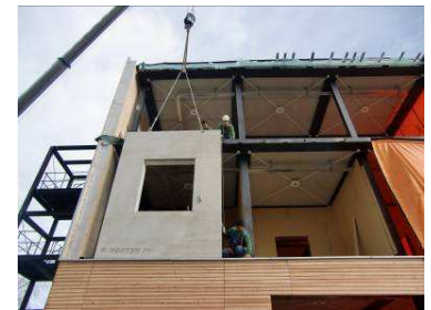
Prefabricated concrete façade element, developed with Norten-pH
