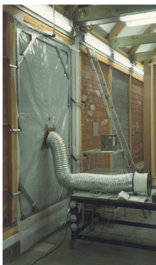
Inside view; an airtightness test is performed on one of the facade elements.
