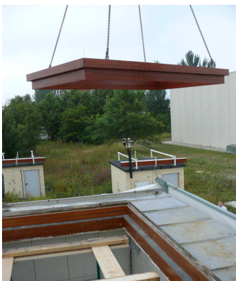
Installing the frame for roof samples in ILARGI.
