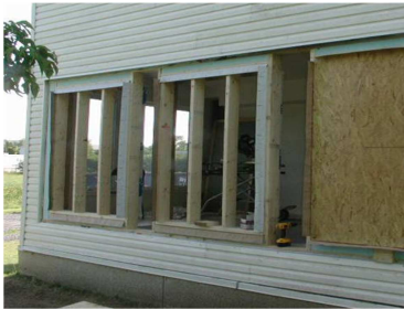
Three test bays in preparation.
