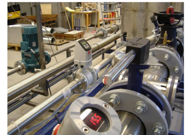
Test of circulation pumps.
