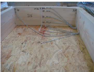
Sensor positioning in a wall assembly
