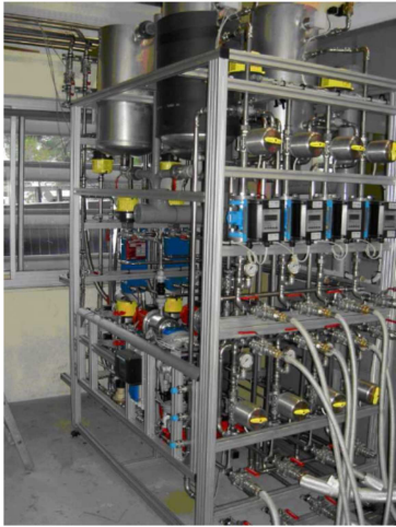
Test bench facilities (High temperature, Emitter and Water drawing modules)
