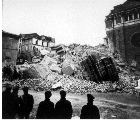
Figure 2-4 – The Civic Tower of Pavia after collapse (Binda et al. , 2000a)
