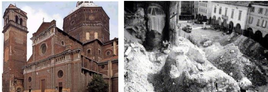
Figure 2-1 – Civic Tower of Pavia before and after the collapse (images from Garavaglia et al. (2006) and Anzani et al. (2009))
