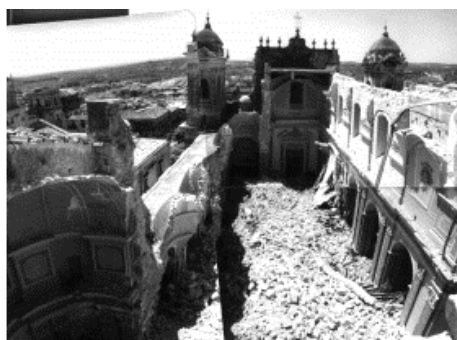
Figure 2-3 – The Cathedral of Noto after the collapse (Binda et al. , 2001)
