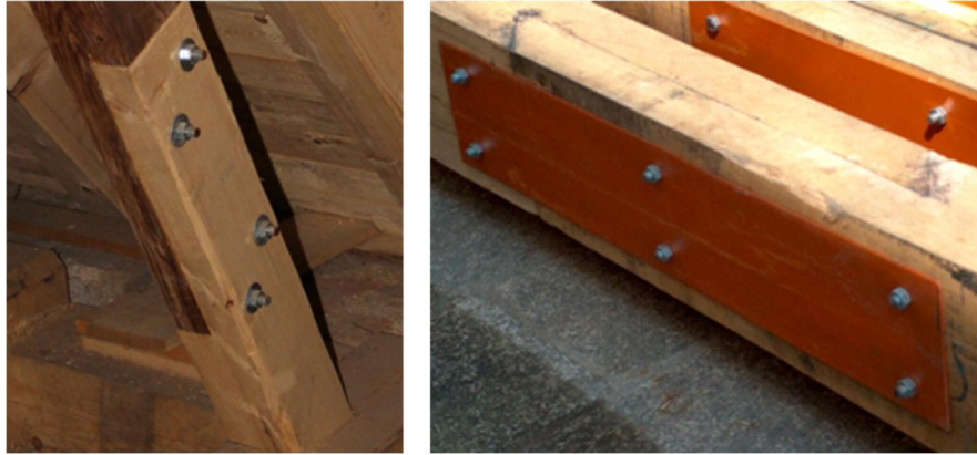
Fig. 22 – Scarf joints reinforced with metal connectors and plates.
