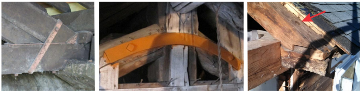
Fig. 16 – Examples of notched joints with metal devices.
