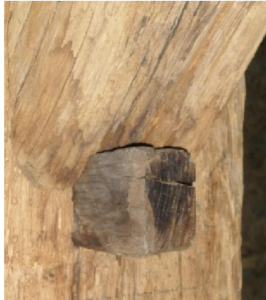
Fig. 10 – Wooden wedge to ensure the contact between the tenon and the mortise.
