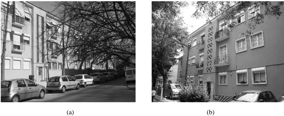
Figure 5.1 Typical masonry buildings in Alvalade neighbourhood, Lisbon.
