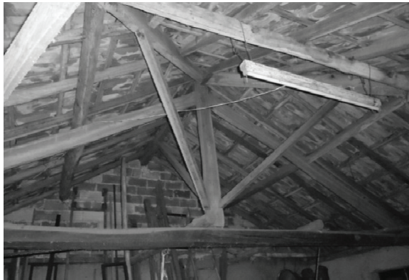
Fig. 16. Covering Structurally Supported by Wood Trusses
