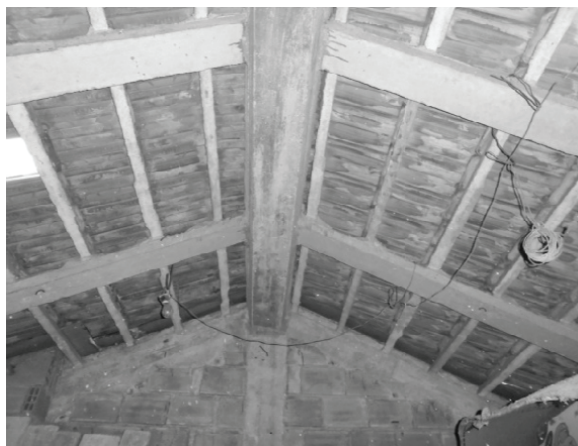
Fig. 17. Covering Structurally Supported by Prefabricated Beams
