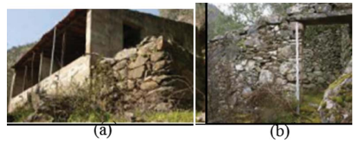
Figure 3. Dwelling houses: (a) house 6; (b) house 55. Credits: Authors.
