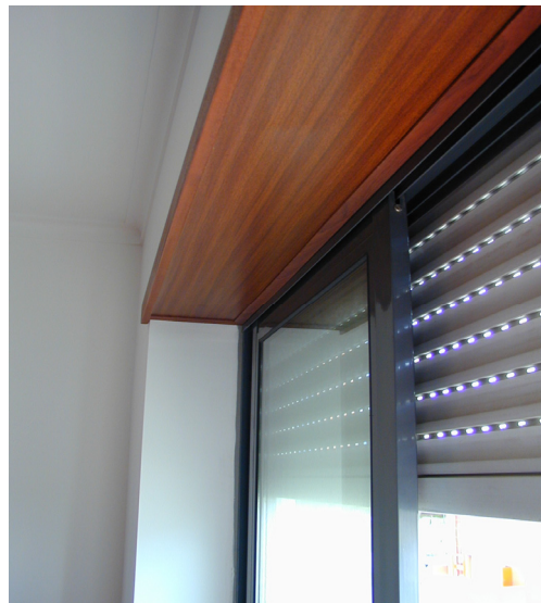
Figure 3 – Cross view of the window tested: shutter SHC
