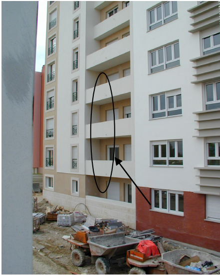
Figure 4 – Building façade (balcony)
