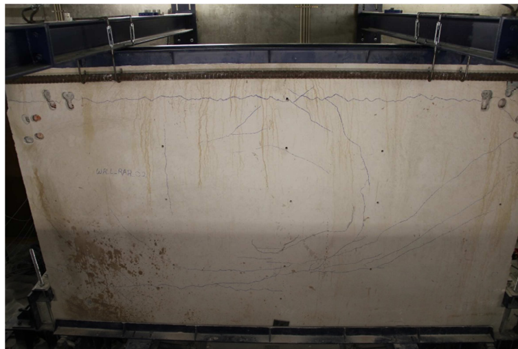
Figure 26: Crack pattern after out-of-plane test
