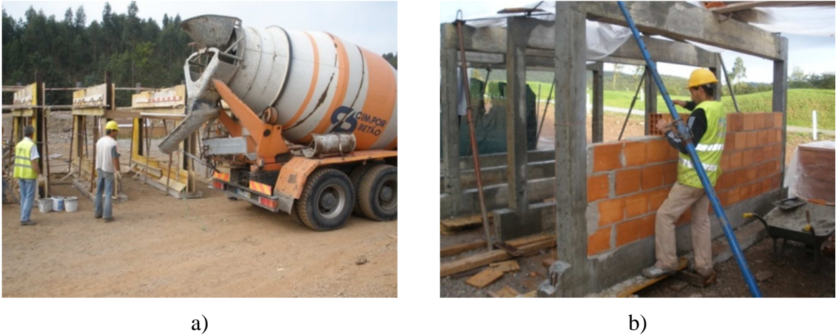
Figure 5: Construction phases of the panels: a) frame concreting; b) wall construction
