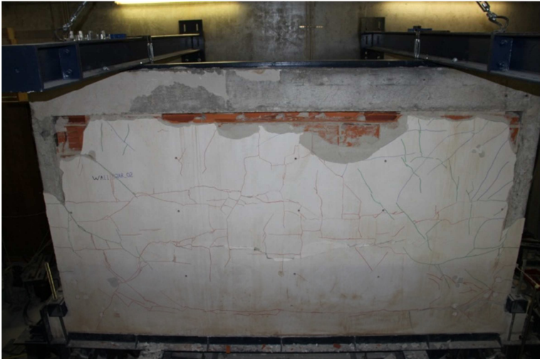
Figure 24: Crack pattern after out-of-plane test
