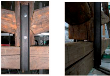
a) UPN profile preventing the out plane movements in the king-post/tie beam connection
