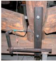
c) Disassemble of king-post/struts joint
