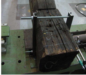
Figure 16: Strengthening of Truss 2 . Screws and binding strip applied in the step front of the rafter-tie beam connection.
