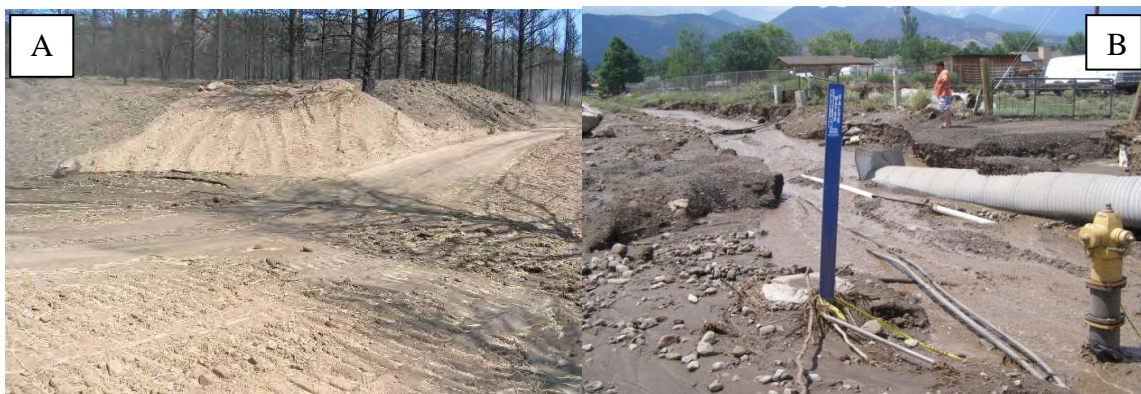
Figure 2. An example of (A) successful culvert removal and construction of low-water crossings on National Forest lands; and (B) a bypassed and breached, undersized culvert on private property, Schultz Fire, Arizona.
