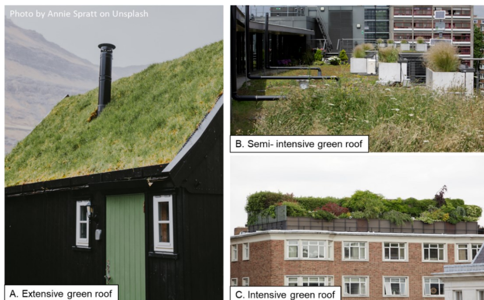
Figure 16. Examples of extensive, semi-intensive and intensive green roofs. Source: Photo (A), credit: Annie Spratt on Unsplash. Photo (B) and (C), credit Imperial College London. Experimental green-roof Eastside, Imperial College London
