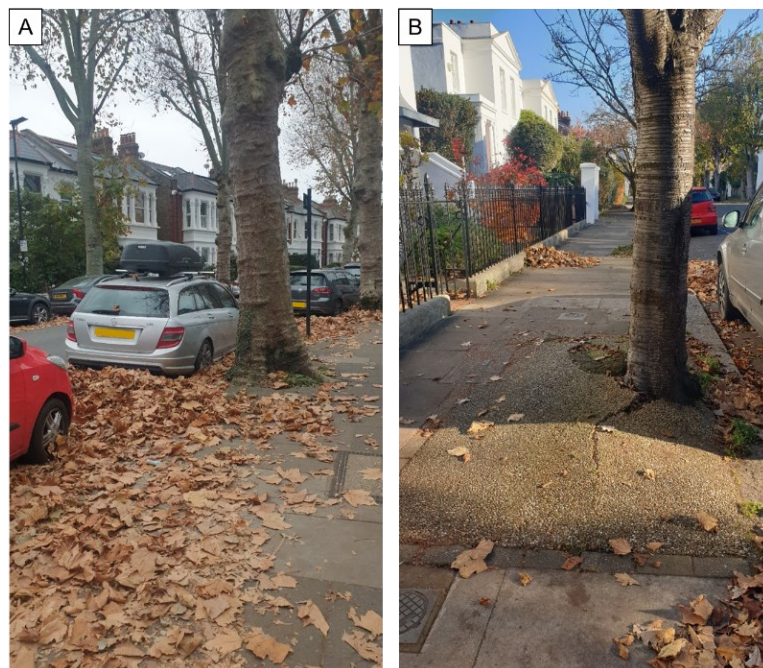
Figure 20. Fallen leaves can become a problem for walking and wastewater systems (A), and tree root growth can cause uneven and broken pavements (B).
