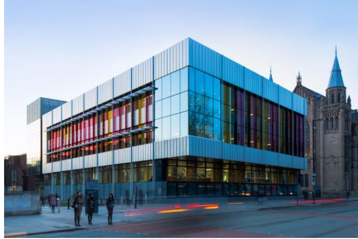
Figure 7.3 Exterior view of Alan Gilbert learning commons
