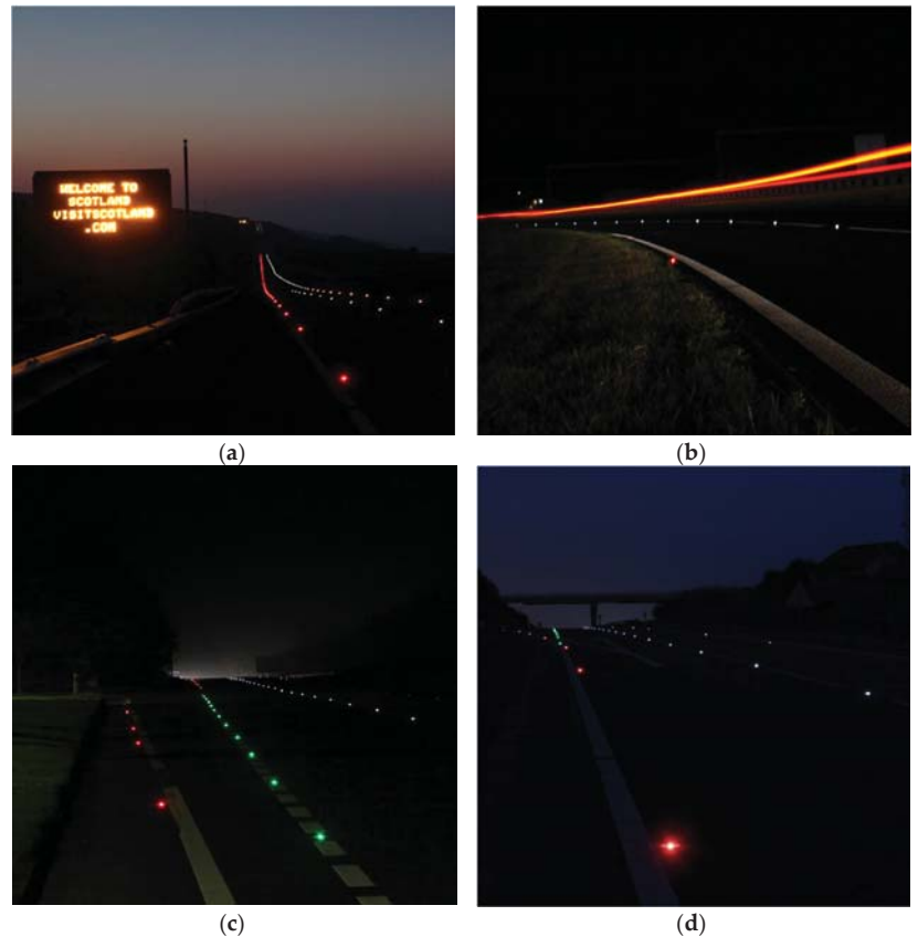
Figure 1. Example active stud installations: (a) dual to single carriageway merge; (b) single carriageway curve; (c) single carriageway junction; (d) dual carriageway junction.
