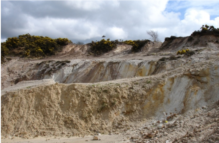
Development works at Hemerdon tin-tungsten deposit. BGS©NERC
