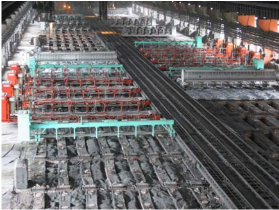
Figure 3: Flue wall condition after years of operation
