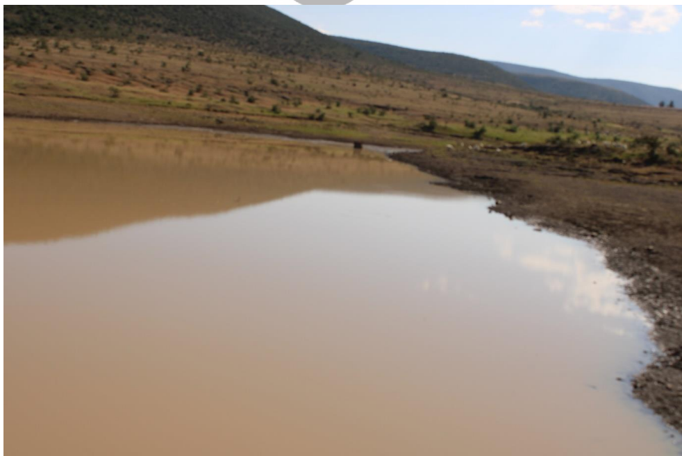
Figure 0.5: Temporary dam constructed in 2012; however, there is no hope for it to be upgraded
