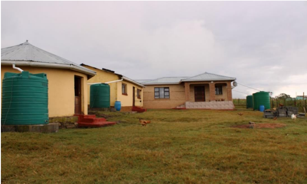
Figure 0.2: Water harvesting tanks installed and are challenged by drought
