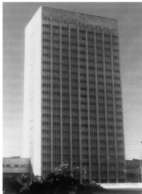
Figure 1 Front view of the 24-floor multispecialty Hermanos Ameijeiras Hospital.
