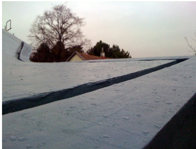
Fig. 5: gutters are completely integrated into the skin
