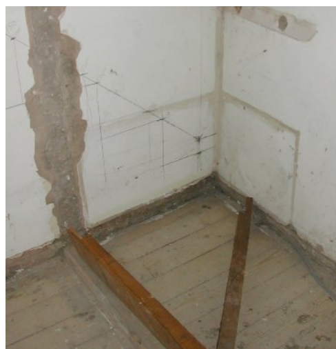
Fig. 2: A 'smooth' space on a construction site awaiting a staircase.
