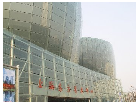
Fig. 6: Close-up of Glass Curtain Wall Photo courtesy of Jinming Ma
