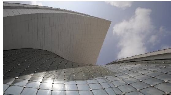
Fig. 10: Close-up of Glass Curtain Wall
