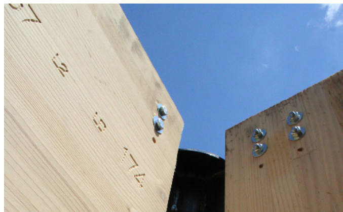
Fig. 9: coded timber panels and different straps
