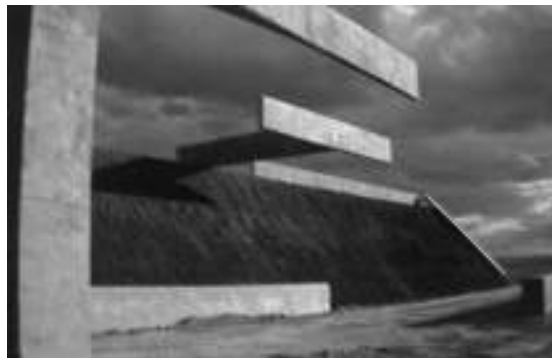
Figure 2.8 Complex City Close up View of the Concrete Extensions
