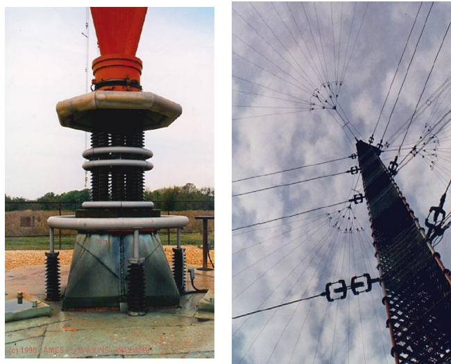
Figure I.11 Isolateurs
