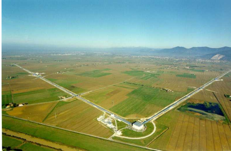
Figure 1. An aerial view of the Virgo gravitational wave detector. The detector Virgo is located in the countryside of Commune of Cascina, a few km south of the city of Pisa, Tuscany.
