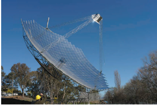
Fig. 16. ANU's 500 m 2 paraboloidal dish concentrator [57].
