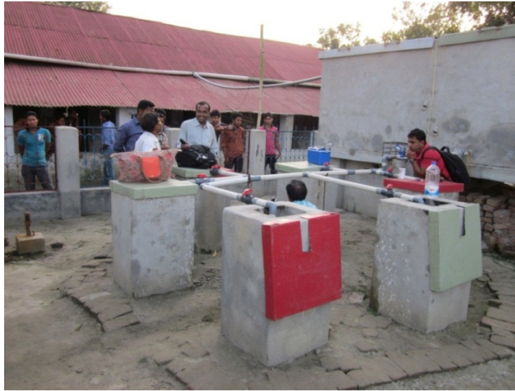
Figure S9: A managed aquifer recharge (ASR) site in southern Bangladesh. A recent intervention, in southwest Bangladesh, to the drinking water salinity problem is ASR. The aim is to store rainwater (with occasional inputs from ponds to meet the functional requirement of the system) in relatively shallow aquifers for dry-season use (Ahmed et al., 2010; Barker, 2013; Hasan, 2012). This approach also has the potential to protect the resource from contamination from storm surges, provided the injection and abstraction wells are capped prior to inundation or staying above the inundation. It therefore provides some resilience against these events. However, its long term sustainability and health impacts are yet to be known.
