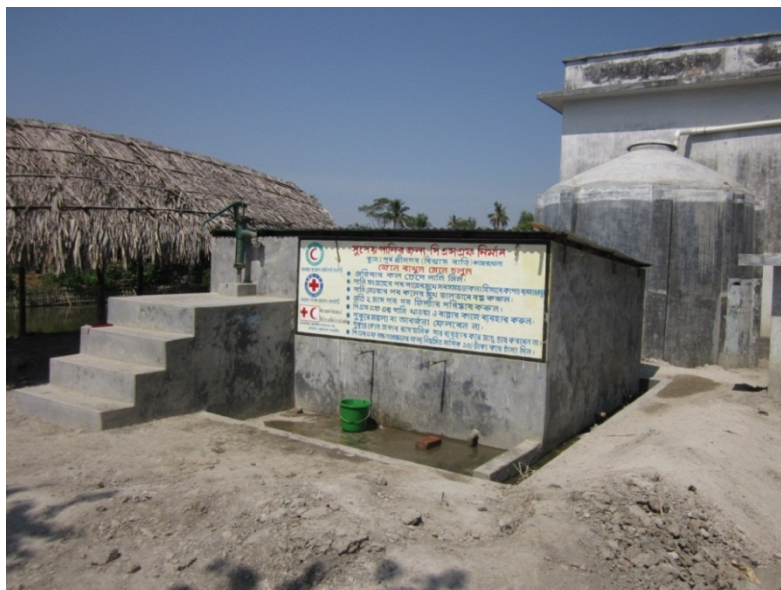
Figure S8: Community base rainwater harvesting and pond sand filter (PSF).
