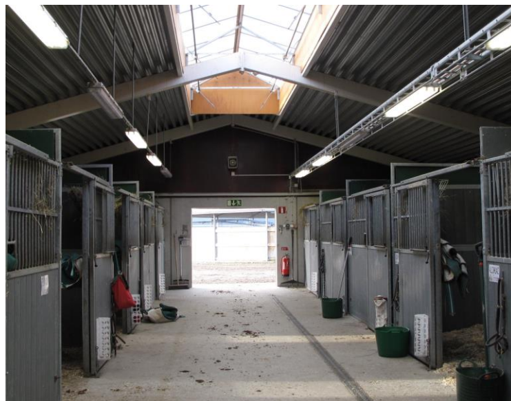
Figure 5. Spacious and bright corridors are important. An example of good safety management practice in horse facilities presented in the InnoHorse web tool. © Christina Lunner Kolstrup.
