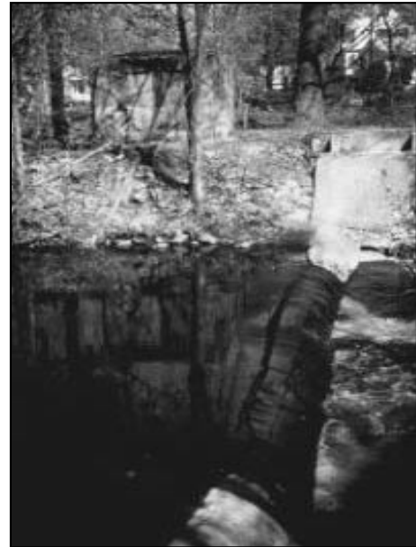
Figure 1. Spreadsheet for computing flood-recurrence intervals showing USGS weir at the Winchester, Massachusetts, gaging station three miles downstream of Woburn wells G & H.
