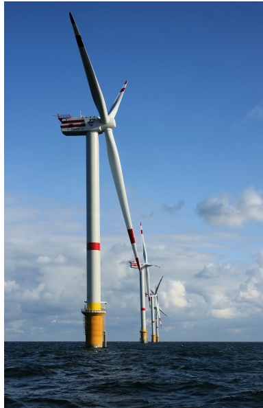
FIGURE 1.1. An example of a Horizontal Axis Wind Turbine. By © Hans Hillewaert, CC BY-SA 4.0, https://commons.wikimedia.org/w/index.php?curid=6361901
