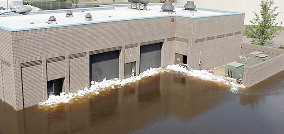
Figure 3. Greenville Utilities water treatment plant surrounded by floodwaters. September, 1999 (Photo courtesy of Greenville Utilities Commission).
