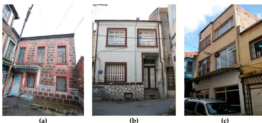
Figure 8. (a) Building 21(HR) (9% energy saving by Package 1; 60% energy saving by Package 2), (b) Building 8 (HNR) (9% energy saving by Package 1; 42% energy saving by Package 2) and (c) Building 11 (C) (44% energy saving by Package 1; 67% energy saving by Package 2) where retrofit solutions can be applied initially.
