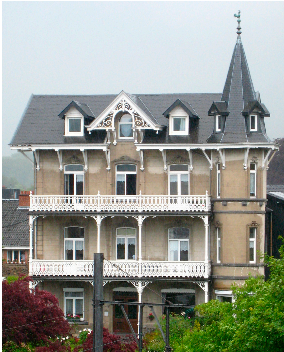
Figure 3. The characteristic features of traditional ‘greatcoat’ architecture, such as wide eaves and hood mouldings, may appear decorative, but their primary purpose is entirely practical: to stop rainwater penetrating weak points of the wall. ©Clive Murgatroyd.
