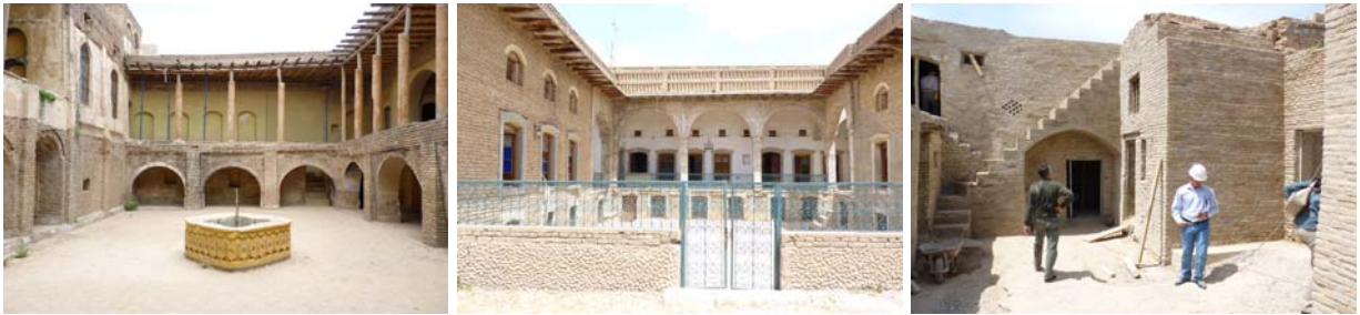
Standing structure in a good state of conservation
