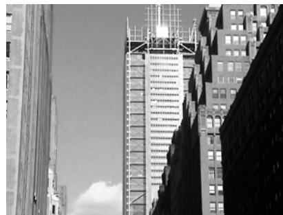
Fig 1. The NYTB during final construction phase. Feb 2007
